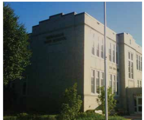
For this budget-neutral program, the District expects to receive over $320,000 in energy rebates/incentives from the NJ Board of Public Utilities Office of Clean Energy and Pay-for-Performance program (P4).
