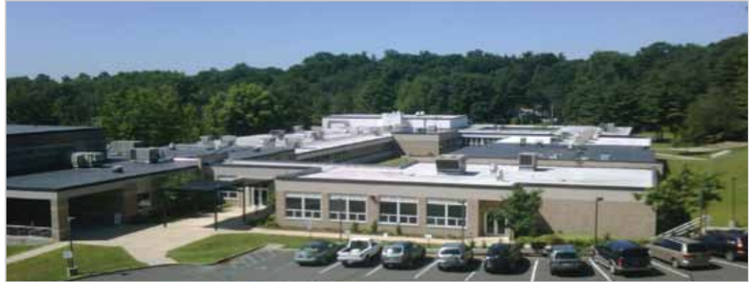
Ameresco took advantage of a new, innovative state program that enables energy cost savings generated from existing budgets to pay for capital, energy efficiency improvements to facilities at no cost to the Somerset Hills School District.
