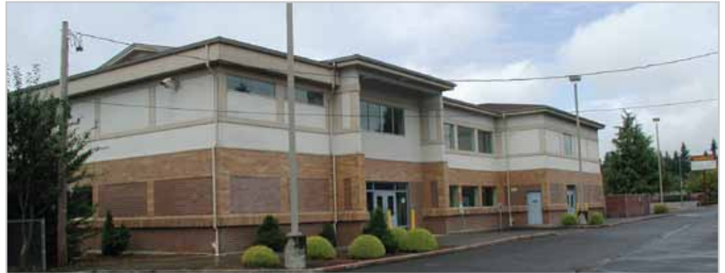
Dating back to 1909, the Battle Ground School District has a proud history serving its communities and now serves 13,000 students in Southwest Washington. Administrators wanted to upgrade the facilities and lower energy and water use.
